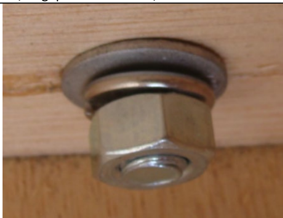
c. Door securing bolt with washer, lock washer & nut
